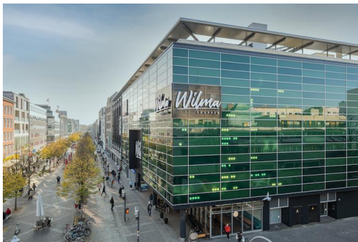
Meeting point in a new design: The modernization of the local supply center has been completed (credit: : Eric Kemnitz / URW)
